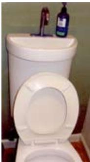
Left: Wash your hands in the sink on the tank lid. The water goes into the tank which has a half or full flush. Greensburg, Top: A Windfarm, old vs new at Spearville, KS.
